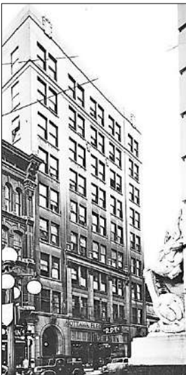
(Left) The Ottawa Electric Building at 56-60 Sparks Street Ottawa, 1950, (subsequently renovated while retaining the façade)
