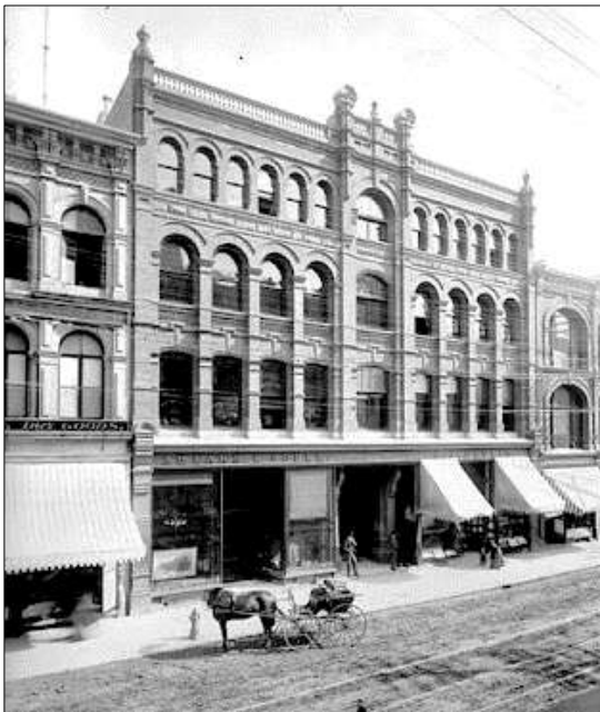
R. J. Devlin & Company Building, 76 Sparks Street, with Ahearn & Soper appliance store (behind parked carriage), 1891.
